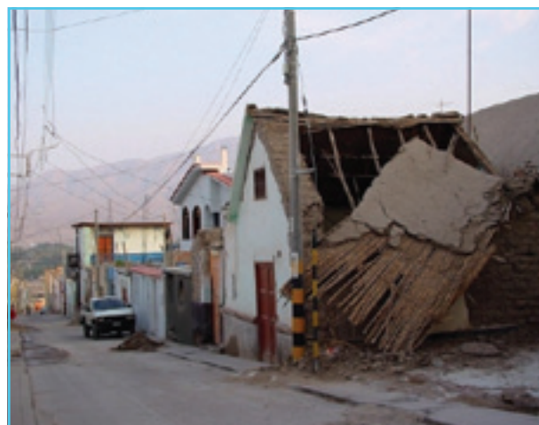
This roof collapsed during an earthquake in Moquegua, Peru, because of poor anchoring to the walls
