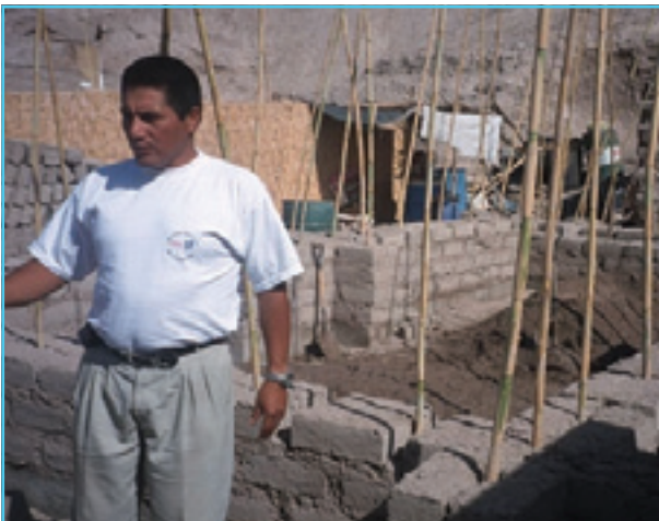
A reconstruction project in Tacna, Peru, where adobe housing had failed in an earthquake. In reconstruction, the quality of adobe production was strictly controlled and walls were reinforced with cane
